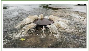
I & I can overload our sewer system causing overflows of raw sewage, reducing the level of treatment at our plant and causing an increase in operating costs.
