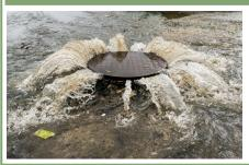
I&I can overload our sewer system causing overflows of raw sewage, reducing the level of treatment at our plant and causing an increase in operating costs.
