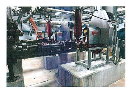
UMJA Staff with the help of R&M Equipment completed the installation of a new Digester blower.
