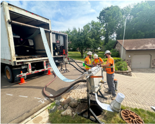
Figure 5. CIPP Liner Installation
