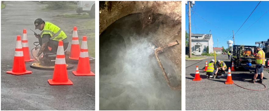
Figure 7. Smoke testing in progress
