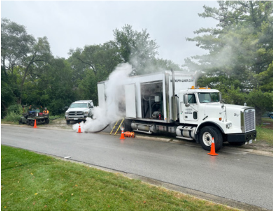
Figure 3. Main sewer CIPP lining
