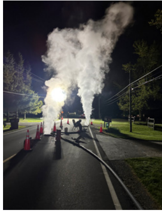
Figure 4. Steam curing CIPP
