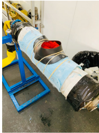
Figure 6. CIPP Lining System
