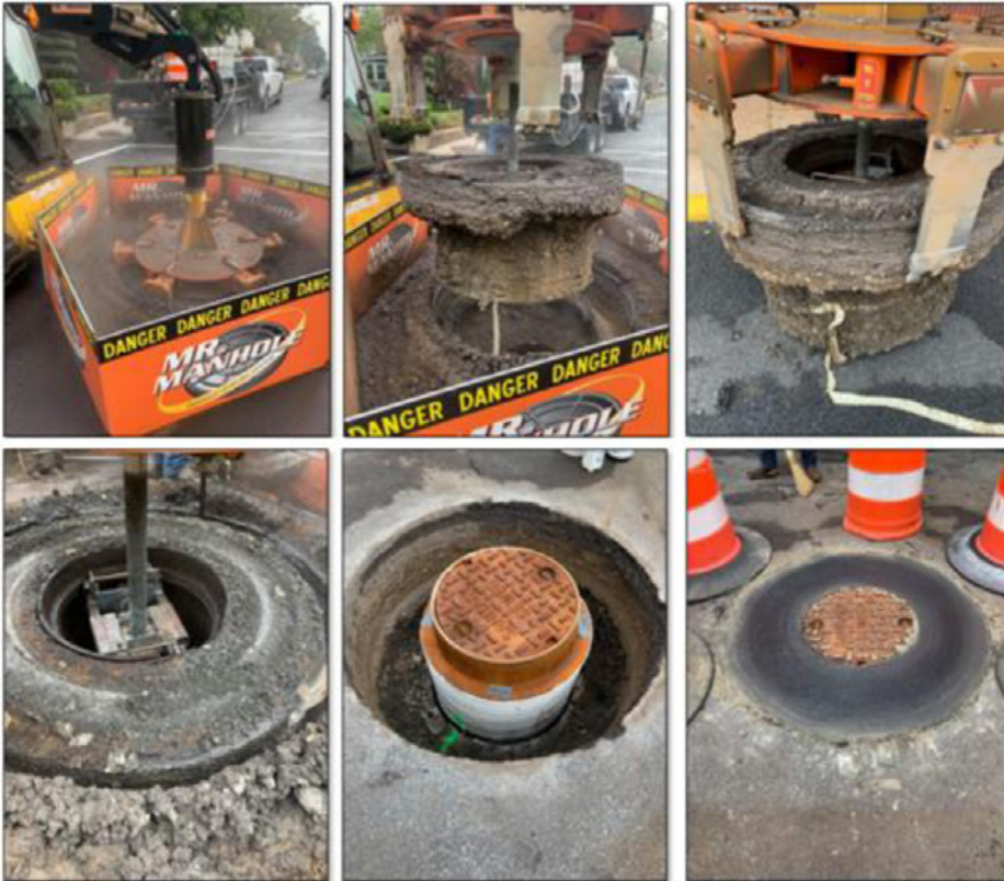
Figure 2. Mr. Manhole Installation System
