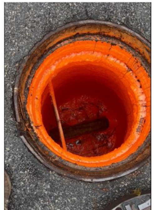
Figure 1. OBIC Composite Polyurea Lining System
