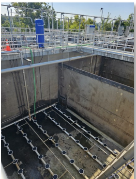
Photos taken after taking tank offline for routine service. Notice a break.
