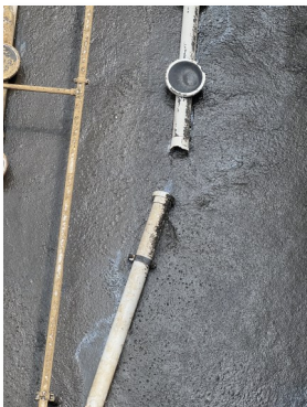
Photos taken after taking tank offline for routine service. Notice a break.
